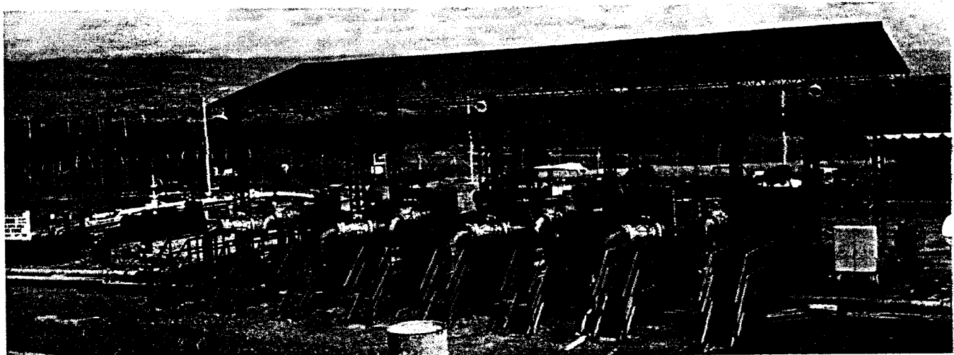
Vibration and pulsation problems at this pump station were improved following analysis of acoustical characteristics of the piping systems and installation of all-liquid filters and modifications to suction piping.
