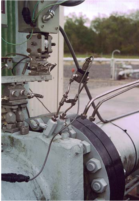
Figure 20 – Differential Pressure Transducer Installed on the Auxiliary Orifice Taps
