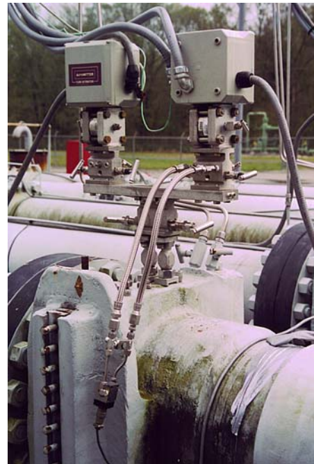
Figure 14 – Temporary Differential Pressure Transducer Installed with Flexible Hoses
