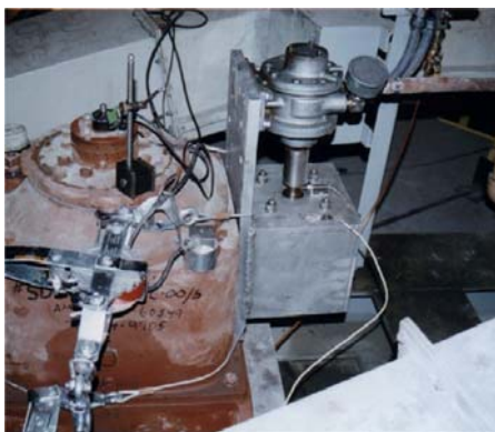
Figure 25: Shaker Temporarily Mounted to Gearbox
