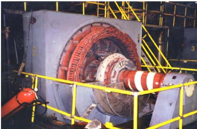
Figure 15: Generator and Bearing Pedestal
