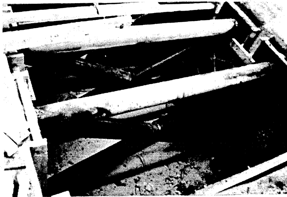
Figure 13: Frames Installed between Foundation Blocks
