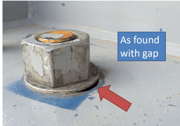
Figure 4. Anchor Bolt at Motor Base
