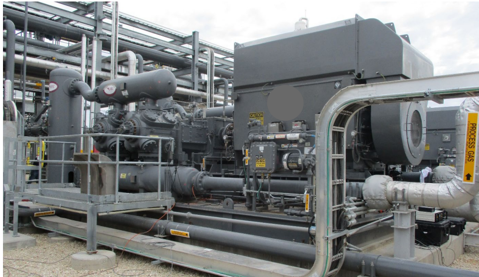
Figure 16. Motor – Compressor Unit
