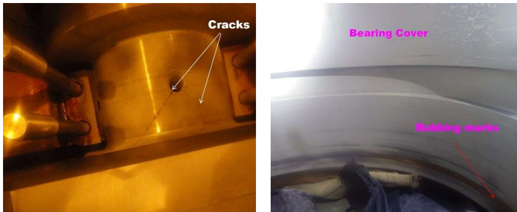
Figure 8 – Compressor crankshaft cracks and bearing damage
