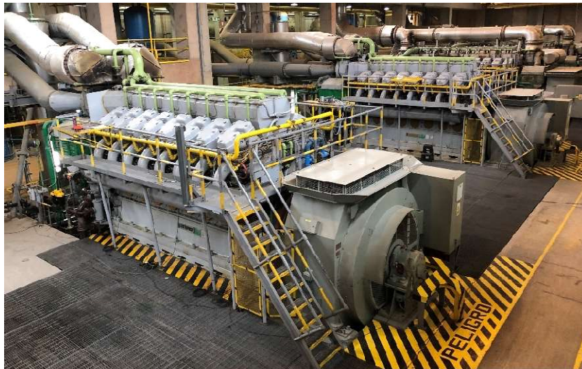
Figure 1. Engine – generator units
