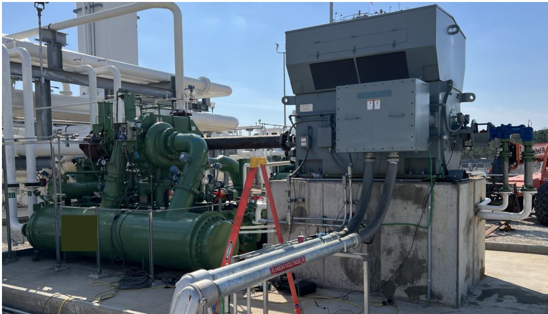
Figure 1 – VFD Motor, Coupling, and Compressor for Unit 2
